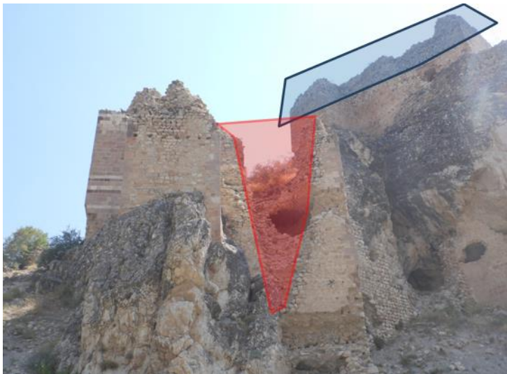
Fig.4. Demolitions in the western side of the castle
